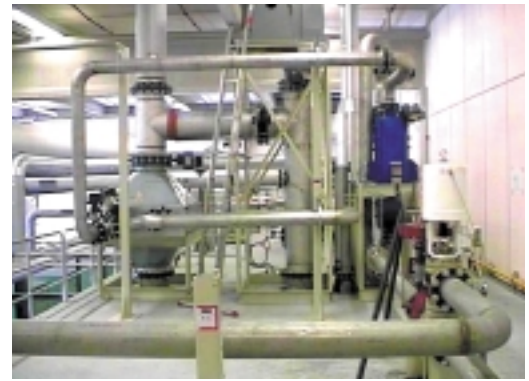
A view of the installation on the mezzanine above the air cycle machine test cell. In this installation, heat exchangers are air-to-outside-air. Liquid heat exchangers are also practical, depending upon local utility costs and supplies. The test system was under construction at the time of this photo.
